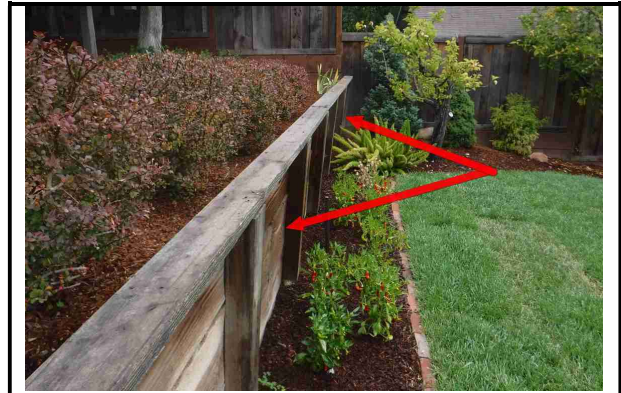
Displaced rear retaining wall.
