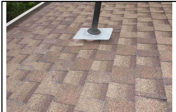
Improperly installed flashing.
