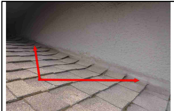
Improper roof-to-wall flashing.
